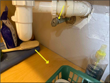
Right bedroom bathroom
