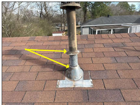
properly position exhaust collar(s)
