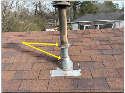
properly position exhaust collar(s)
