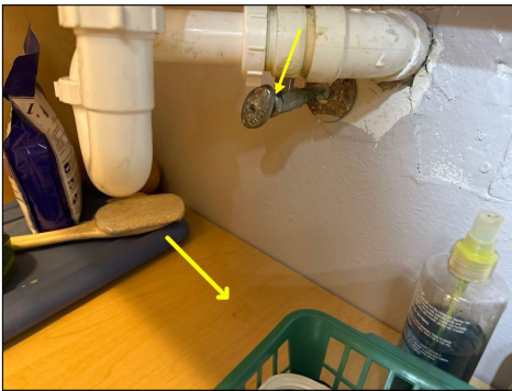
Right bedroom bathroom
