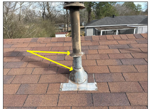
properly position exhaust collar(s)
